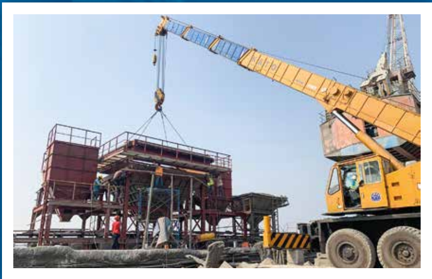
Mongla Cement Factory : Fabrication, Erection & Commissioning of 01 No. Eco Hopper.
